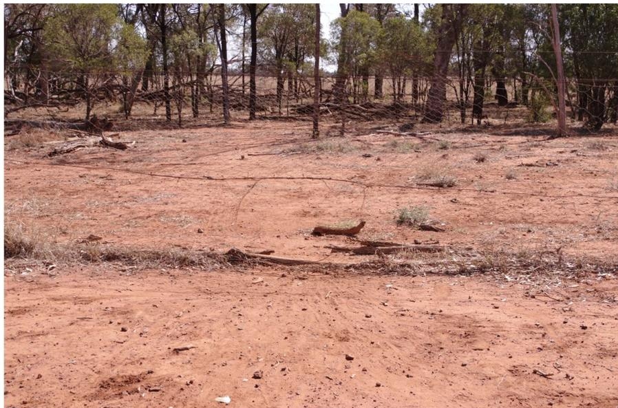
*Figure 6. Vermin fence in disrepair at Morven, with holes large enough for easy passage of sheep, goats, macropods and wild dogs*
